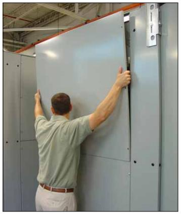
Figure 40. Tilting the Cover Away from the Frame.
